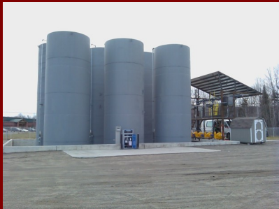
Dead River Bulk Facility Built by FPH—2009
